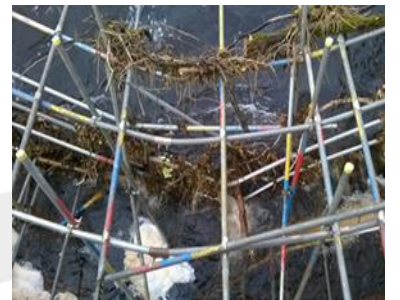
On site showing bent tubes
