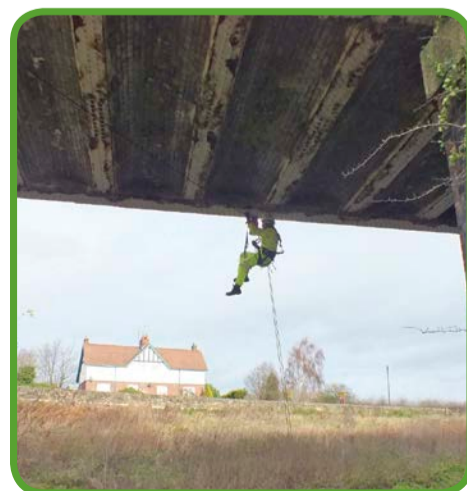
Bridge inspection and assessment, Derbyshire
