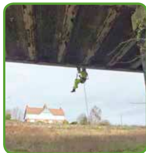
Bridge inspection and assessment, Derbyshire
