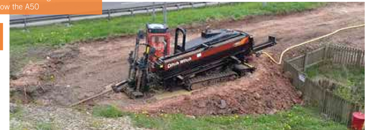
Directional drilling services below the A50
