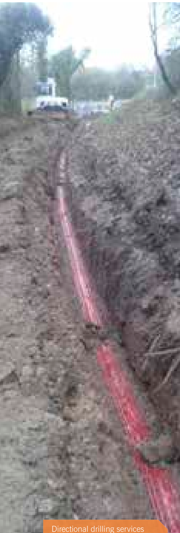
Directional drilling services below the A50
