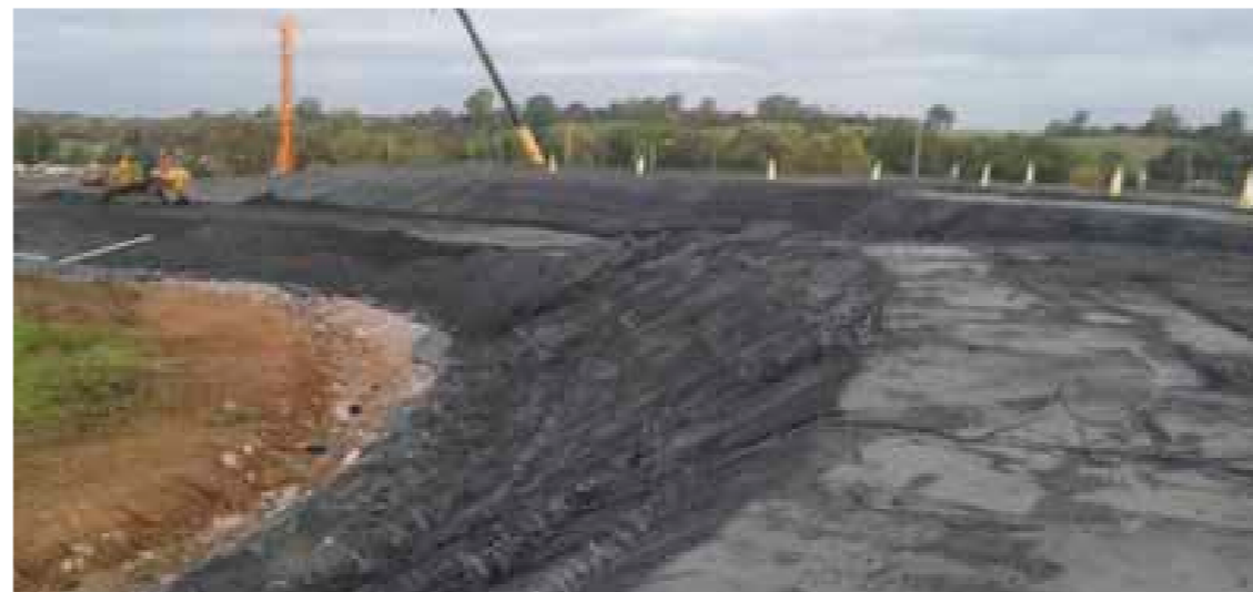
Lightweight PFA used for the main embankments
