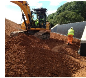
Class 1A material being placed and compacted
