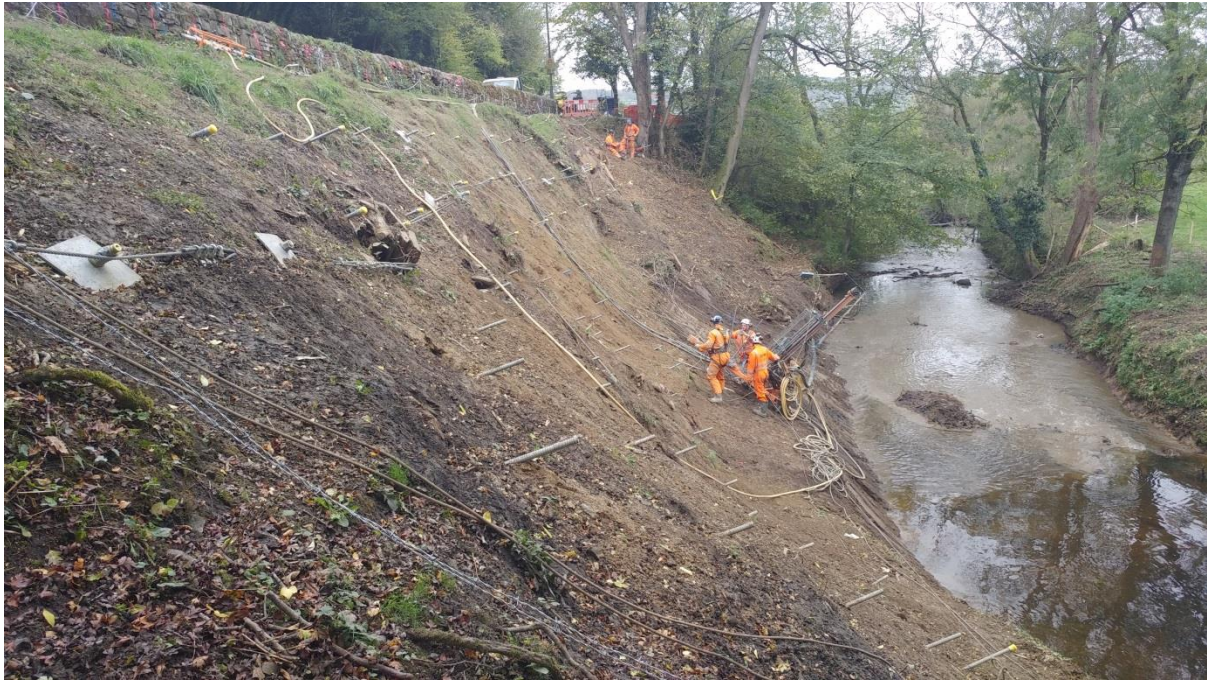
Figure 9 – Whole Site during Construction
