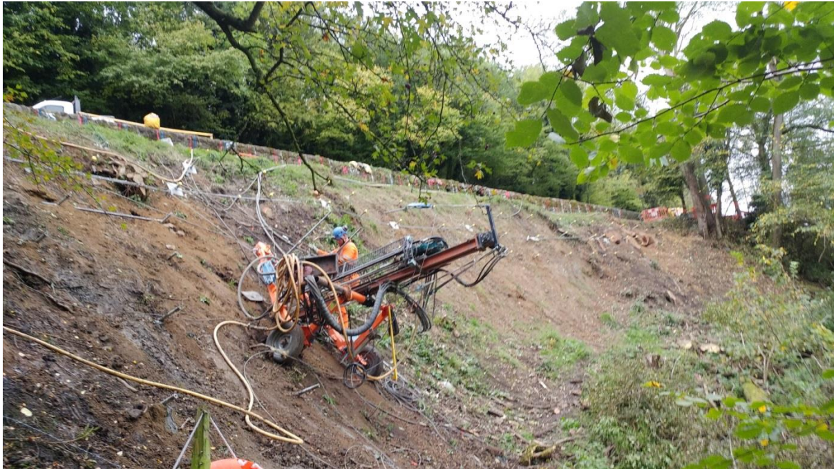
Figure 8 – Soil Nailing using Roped Access Techniques
