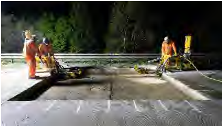
Full depth repair + drainage!
