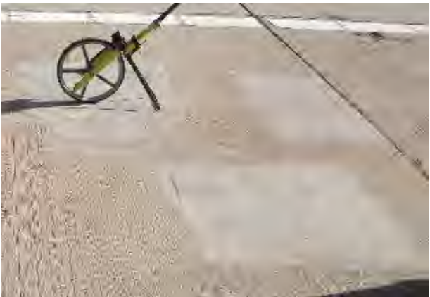
Thin bonded and shallow repair
