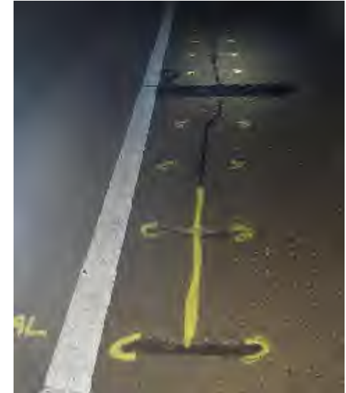
Crack stitching
