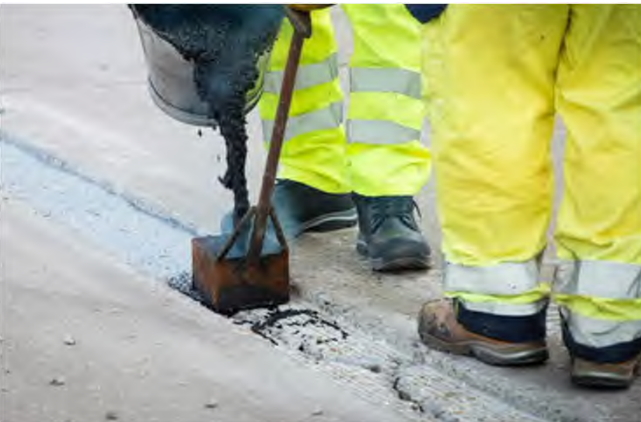
Inlaid crack repair
