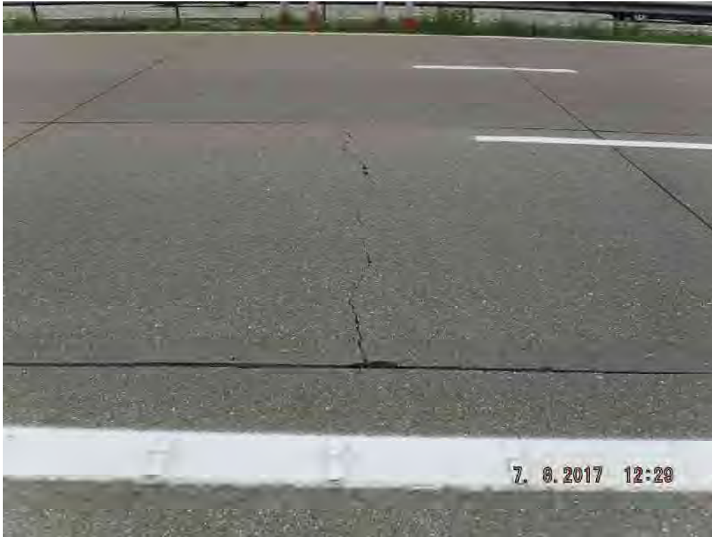
Transverse crack
