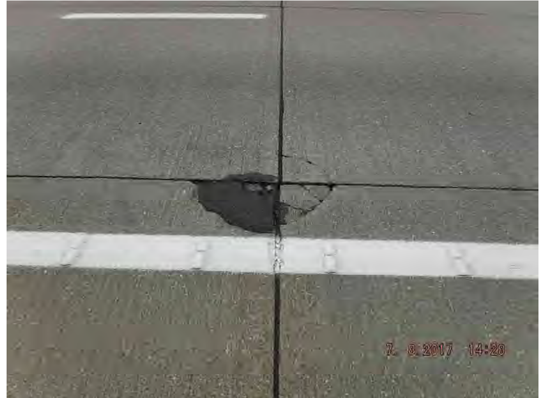
Corner crack
