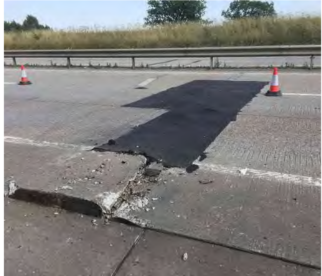
Compression failure or 'blow up'
