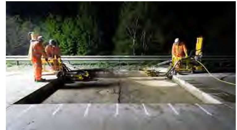
Full depth repair + drainage!
