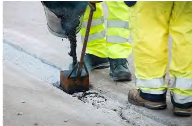
Inlaid crack repair
