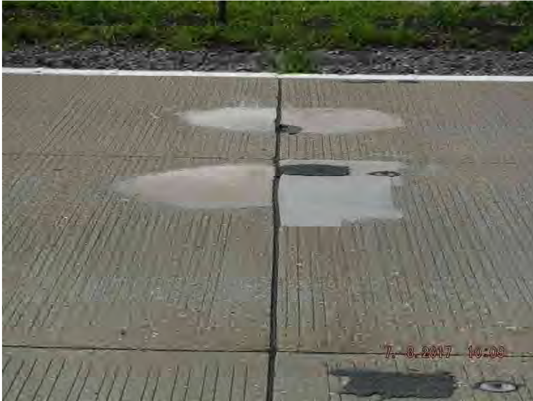
Deep joint spall
