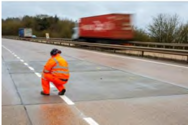
National Highways Concrete Pavement Asset Management and Whole Life Cost
