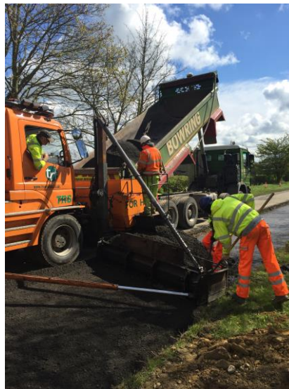
Haunching & Edge strengthening
