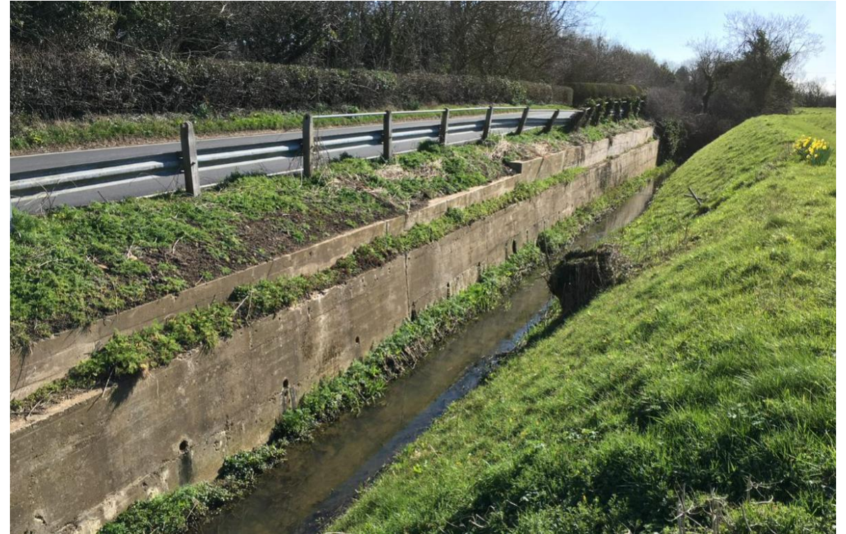
March 2023 site photo
