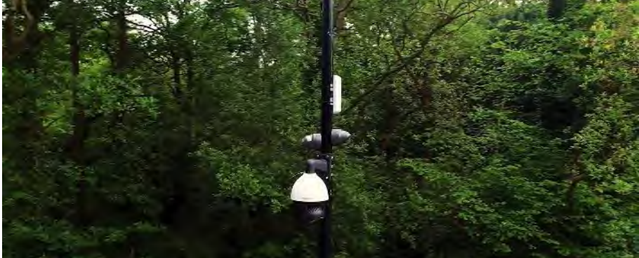
River Shannon Greenway at University of Limerick – 4m columns with highly focussed lighting that restricts light spill into the trees.
