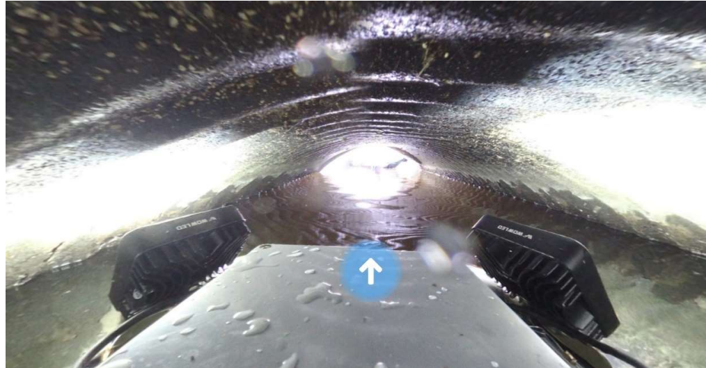
Image through the culvert from ROV camera.
