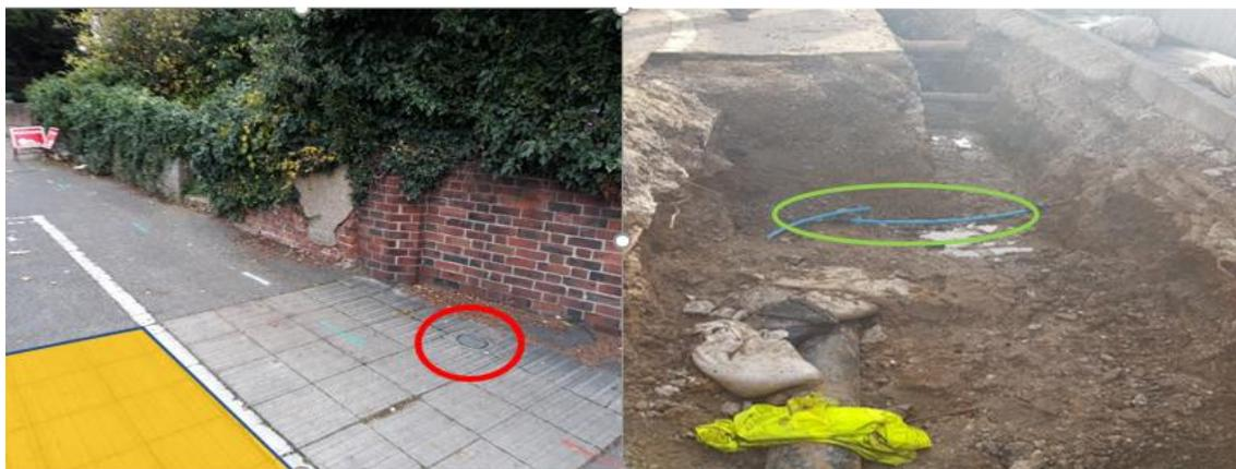
The importance of the water valve is that this was not picked up and highlighted at a number of stages throughout the planning of the works and this was a key significant finding leading to the damage.
