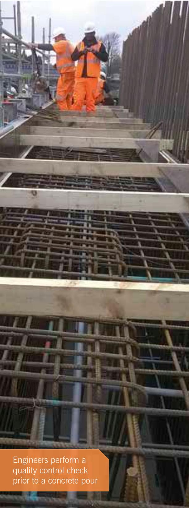
Engineers perform a quality control check prior to a concrete pour
