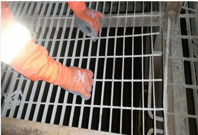
How the floor was originally.
