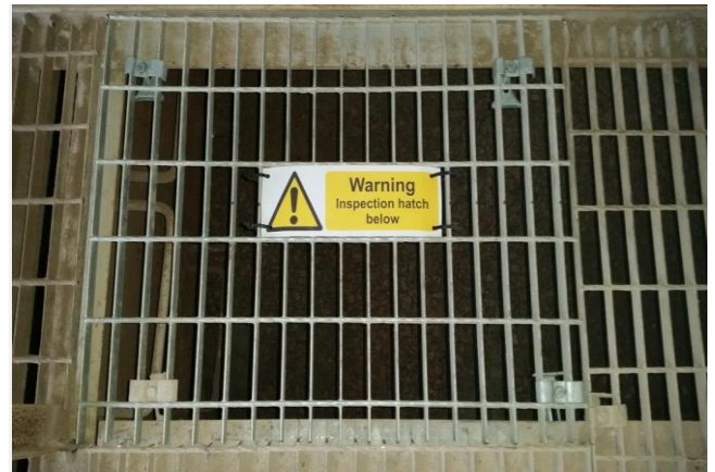
New section of floor.
