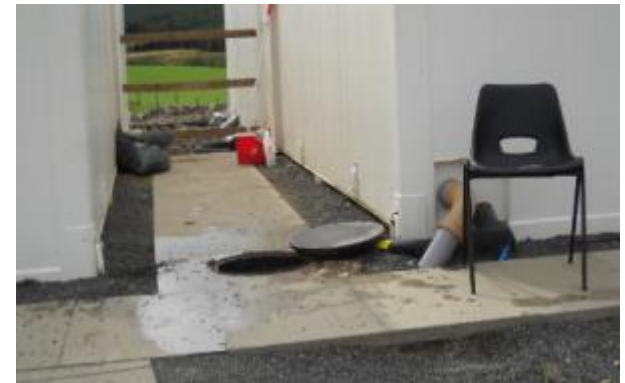
INSPECTION CHAMBER AT ACCESS 1 WELFARE AREA (Post -incident)
