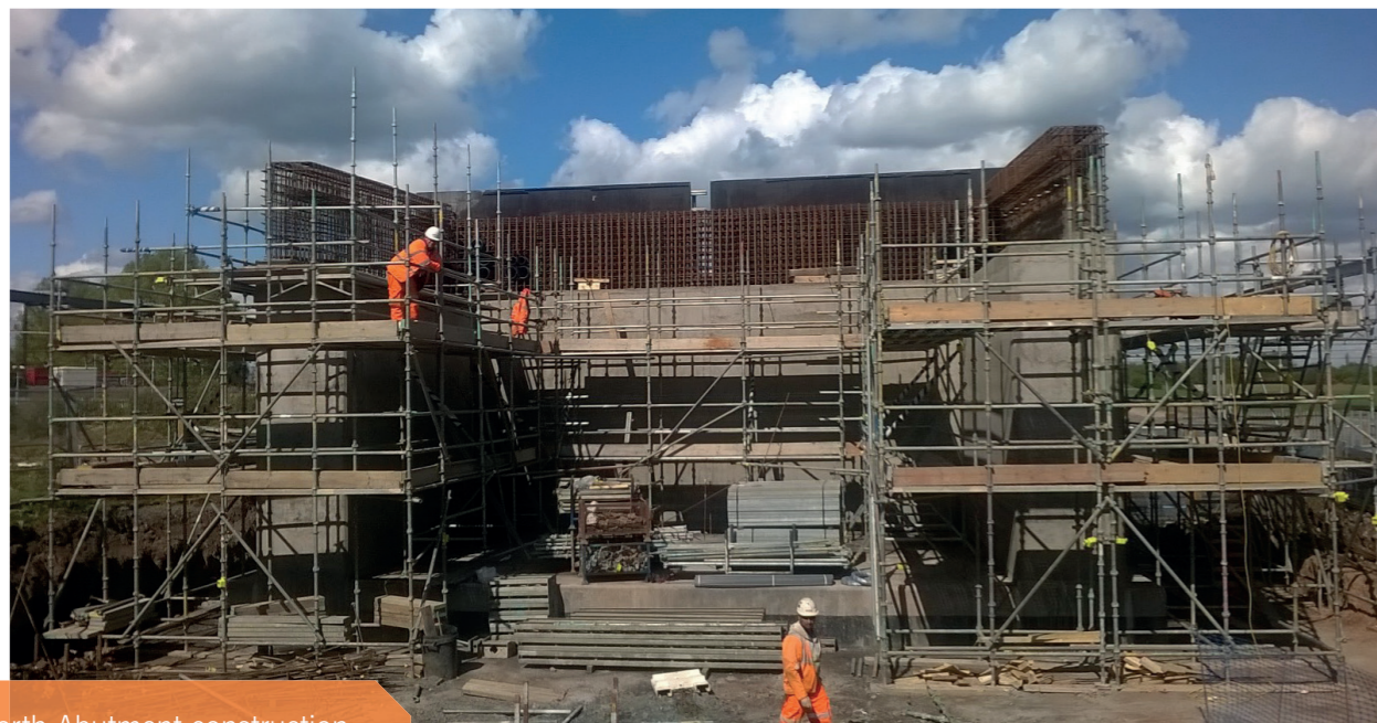
North Abutment construction
