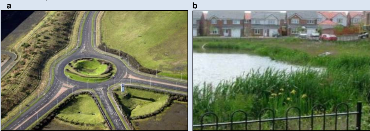
Figure 11: a) Detention basin DEX Roundabout (University of Abertay/SUDSNET) b) Pond at Dex (Scottish Government)
