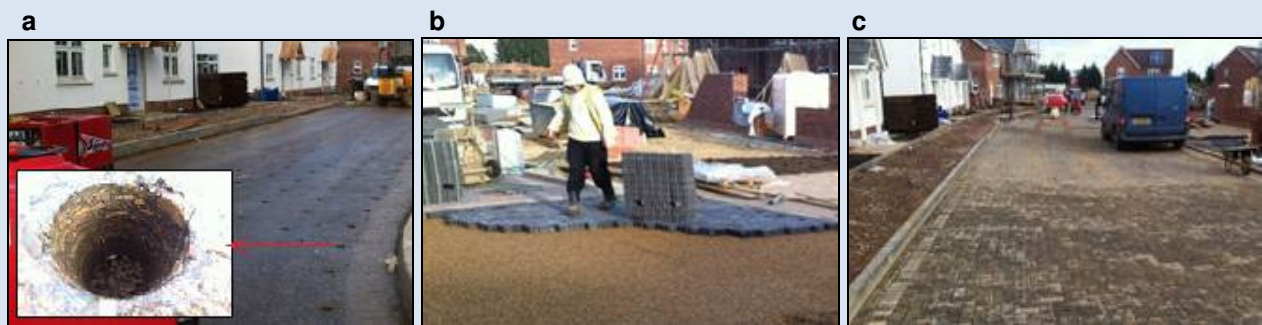
Figure 9: Permeable paving construction stages
