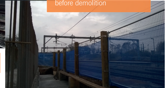
Bridge No. 98 over the West Coast Main Line (WCML) before demolition
